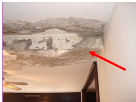
Photo 1 – Appartement R+1 - AVIT
